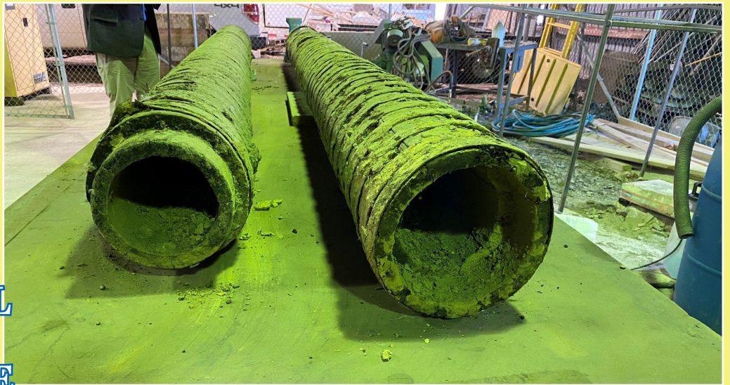
Wooden water pipes that were discovered at ERDC, showing how the pipes would connect through a male and female connection. Photo by W. Andy Martin.
