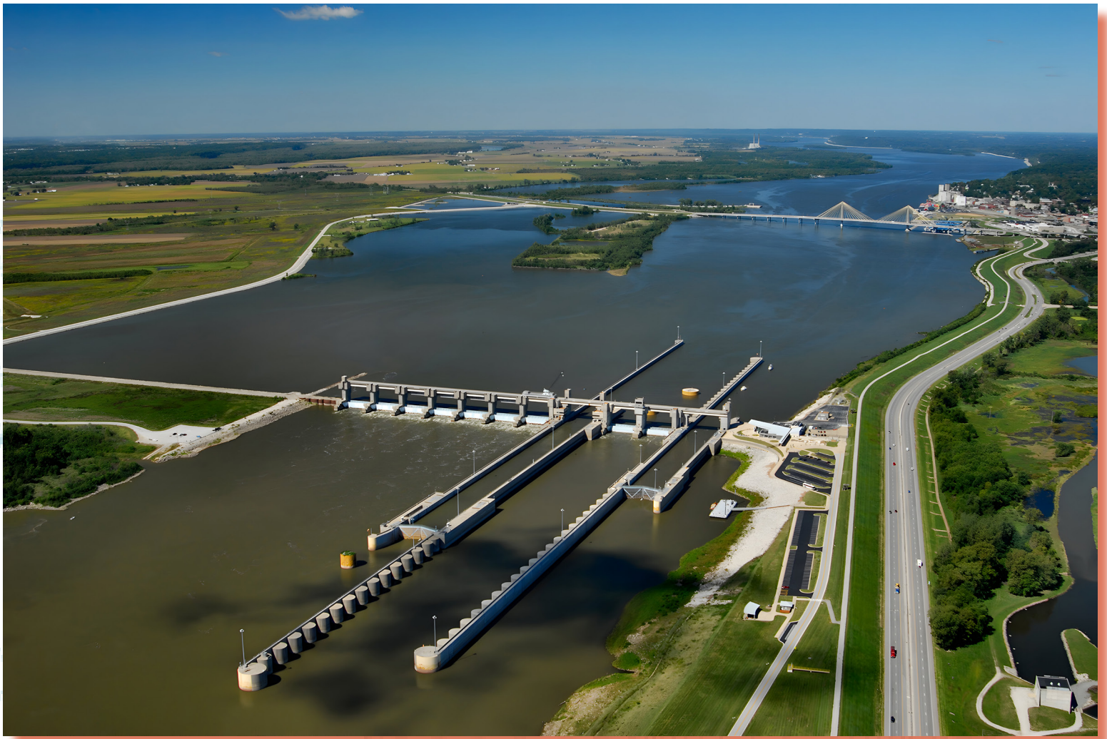
Melvin Price Locks & Dam located on the Mississippi River. Photo courtesy of USACE Mississippi Valley Division Public Affairs Division
