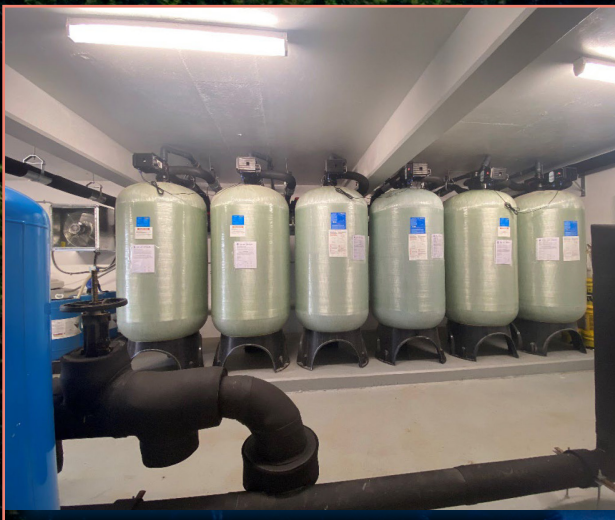
Left: GAC tanks area. Middle: A waterline is installed at Bucks Harbor to bring clean drinking water to residents. Right: The contractor digs a trench to run the waterline. Photos courtesy of USACE.
