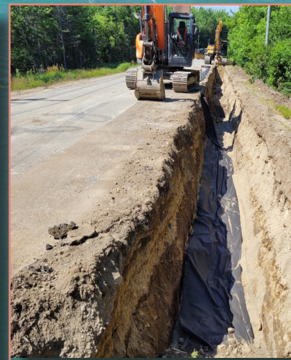
Left: GAC tanks area. Middle: A waterline is installed at Bucks Harbor to bring clean drinking water to residents. Right: The contractor digs a trench to run the waterline. Photos courtesy of USACE.
