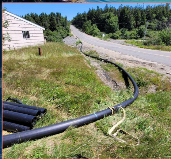
Left: GAC tanks area. Middle: A waterline is installed at Bucks Harbor to bring clean drinking water to residents. Right: The contractor digs a trench to run the waterline. Photos courtesy of USACE.
