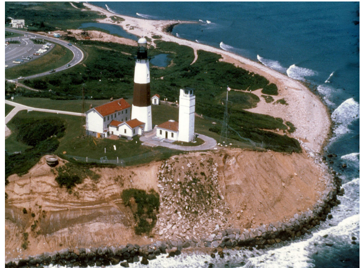
Eroding cliff The eroded cliffs at the Montauk Point Lighthouse in 1968.
