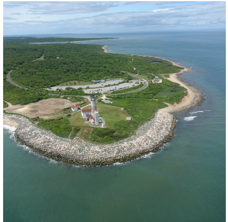
Completed Montauk Point Coastal Resiliency Project.
