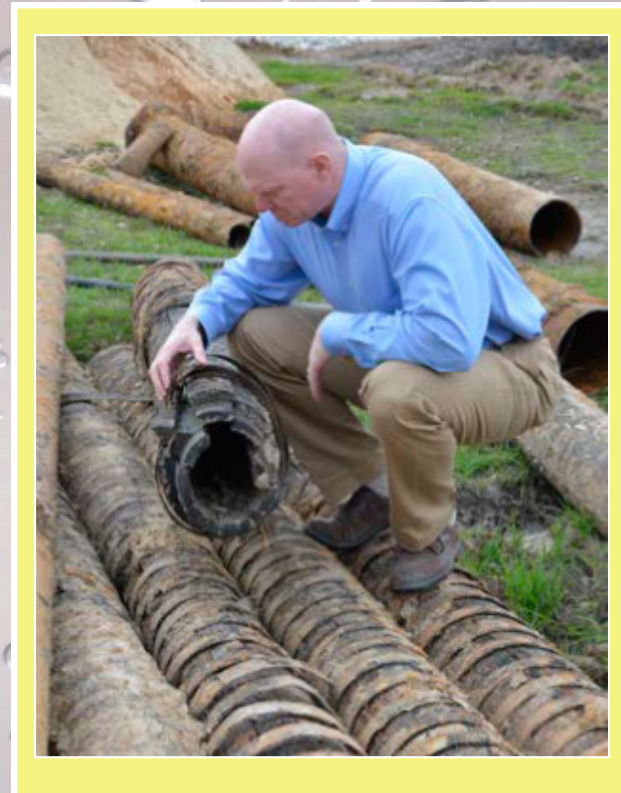
Mr. Craig Prevost inspecting the wooden water pipes that were discovered at ERDC during recent excavation work. Photo courtesy of ERDC PAO.
