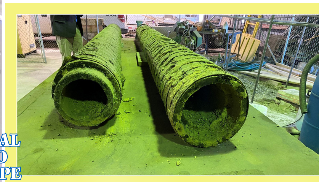
Wooden water pipes that were discovered at ERDC, showing how the pipes would connect through a male and female connection. Photo by W. Andy Martin.
