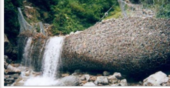
1. Debris flow netting
